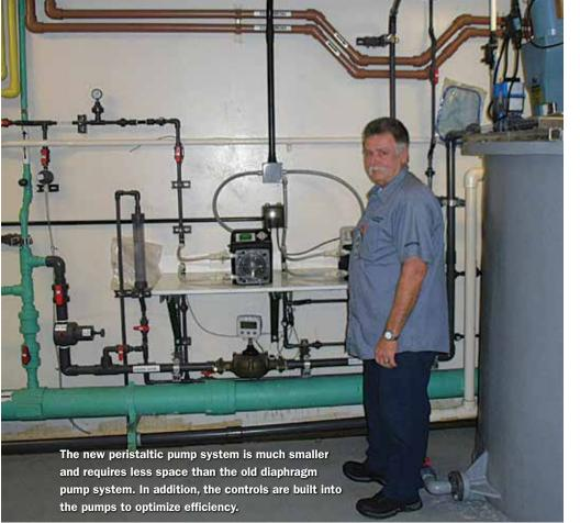
The gas system is expensive to maintain, costing \$10,000 per year for scrubber and injector cleaning and maintenance. Using lower-concentration liquid chlorine and UV technology will help the plant maintain lower trihalomethane (THM) levels. The new liquid chlorine system, which uses peristaltic pumps, will be installed in the chemical room. When the gas–chlorine system is removed, the area will be transformed into a much-needed workshop.
