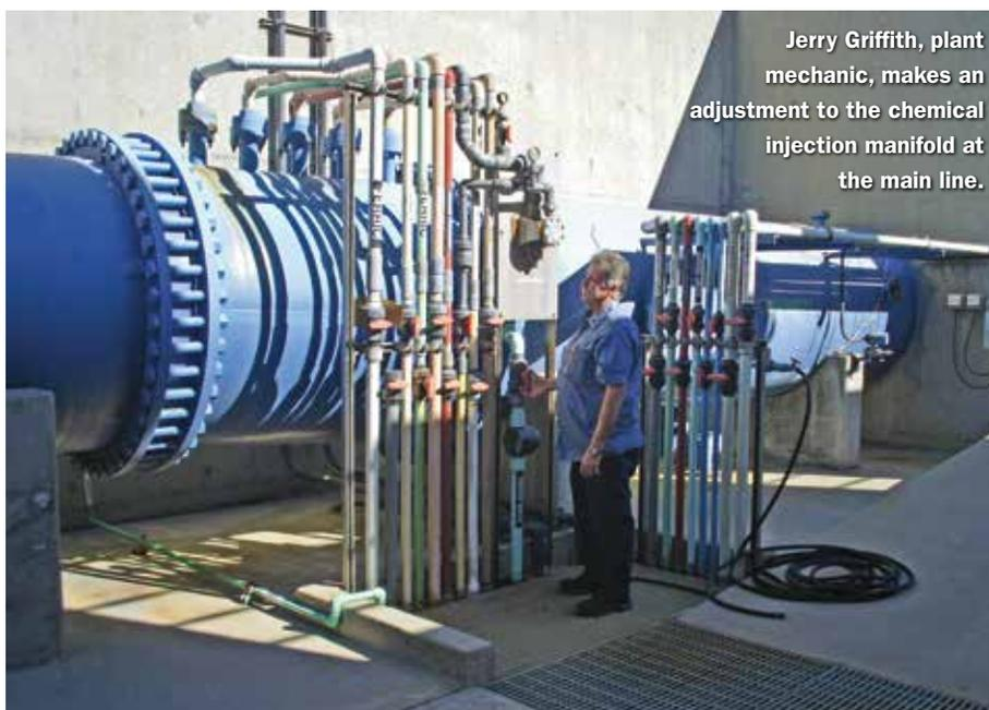
Jerry Griffith, plant mechanic, makes an adjustment to the chemical injection manifold at the main line.
