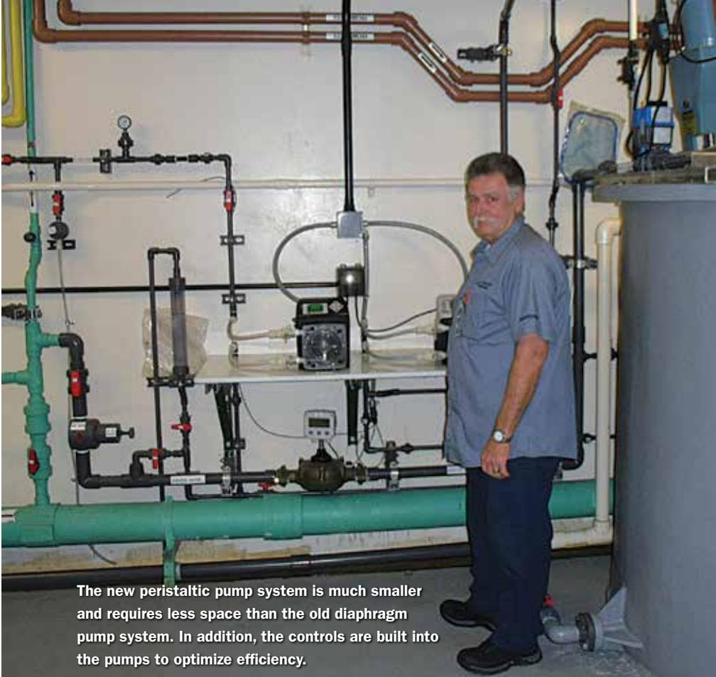
The new peristaltic pump system is much smaller and requires less space than the old diaphragm pump system. In addition, the controls are built into the pumps to optimize efficiency.
